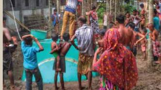
Fiberglass biogas plant installation in progress
